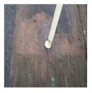
Carefully observe the speed the material is filling the hole, release the pressure from the tubes as you fill to the top of the sleeper.
