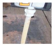
Insert the end of the mixing tube into the hole to be filled and squeeze the trigger to force the material through the mixing tube into the hole. Fill the hole from the bottom upwards, if you start filling from the top only, voiding may occur and you will not get a solid fill.
