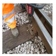
When Spikefast has completed its curing time, it is then ready to drill. The filled hole should be drilled as you would on a new sleeper. If baseplates/chairs have to be adjusted for track alignment, you can drill half and half as in the above photo.
