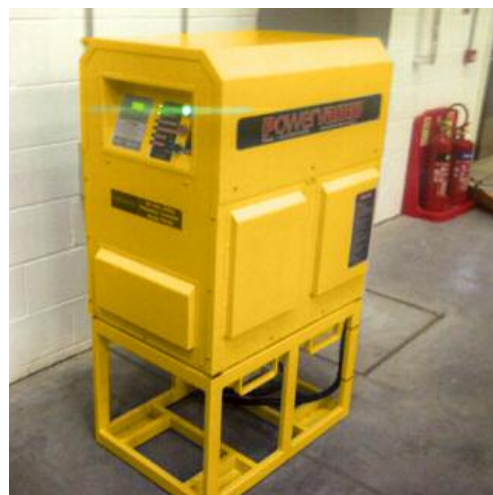
40 kVA fixed hangar power
