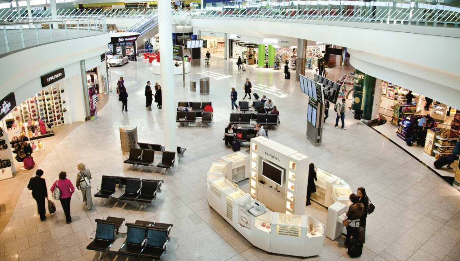
Full Effekta installation of emergency lighting system, Dublin airport, Terminal 2
